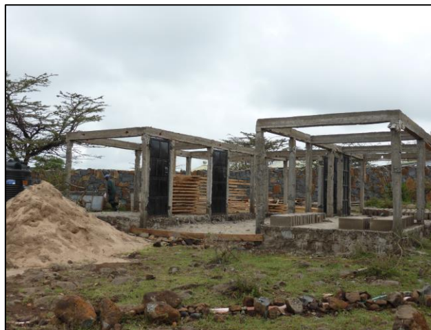
Figure 8: New staff housing being built at the Tony Lapham Predator Hub
